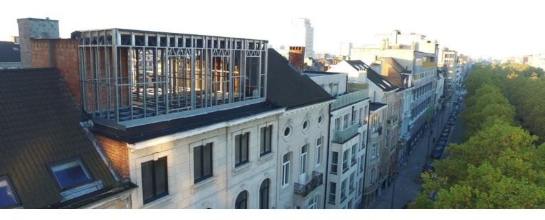
An elevation refers to increasing the height of a building's exterior from the ground level up. One way to approach elevation in construction is through light steel frame construction.
